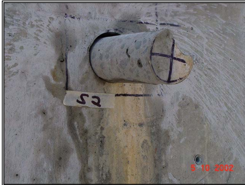
Core S2 was extracted at the tie pin on wall 1.
